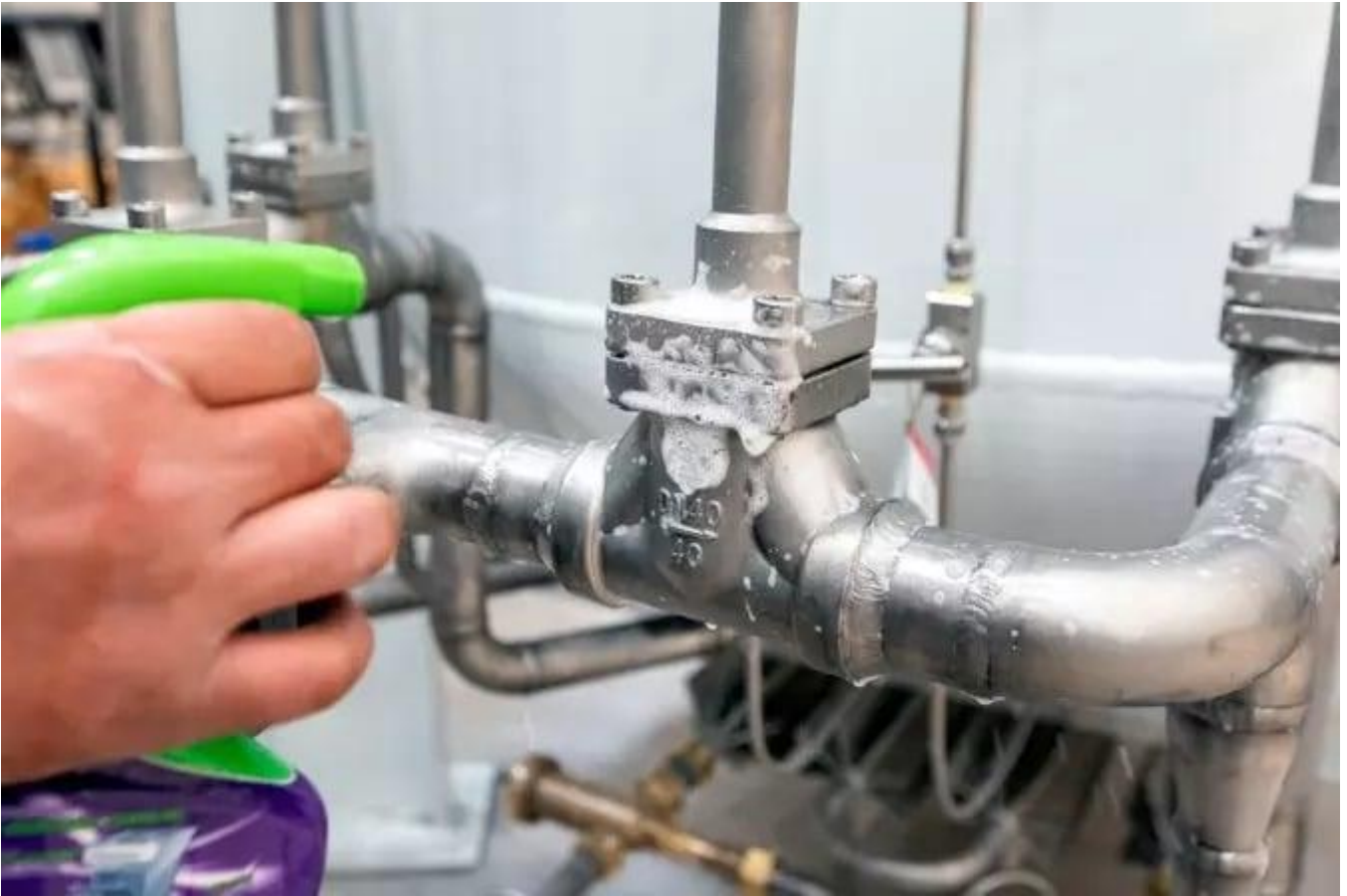
Figure I.14: Leak testing
