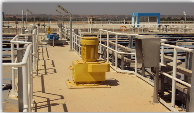
Figure. II.5 Agitateur lent (flocculation)
