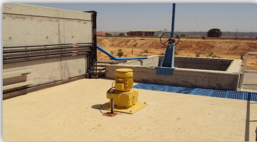
Figure. II.4 Agitateur rapide (coagulation)
