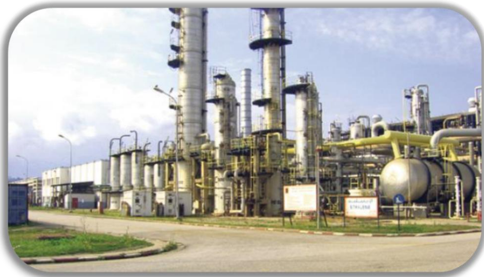
Figure 20 : zone de process
