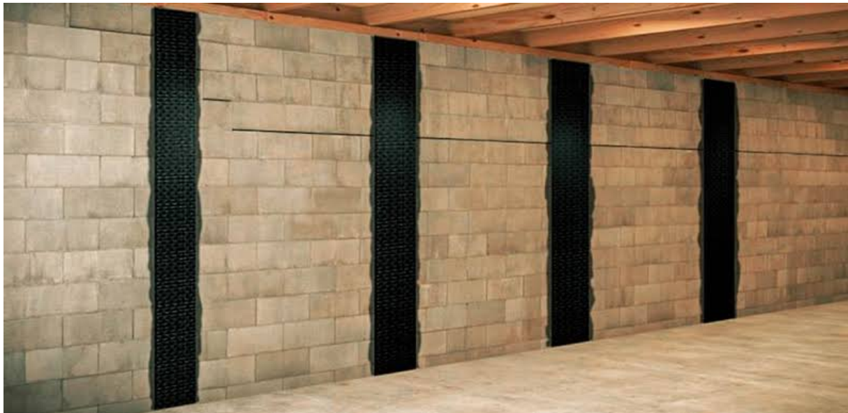
Figure II.6 : Renforcement des murs
