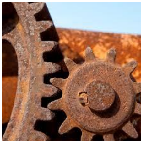
Figure 2.6: La corrosion uniforme
