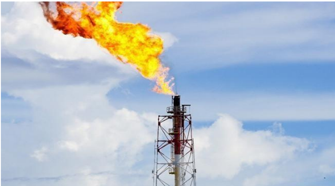
Figure II.1: Torchage du gaz.
