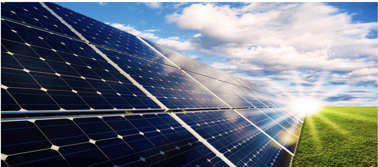
Figure I-1 : installation solaire photovoltaïque [1].
