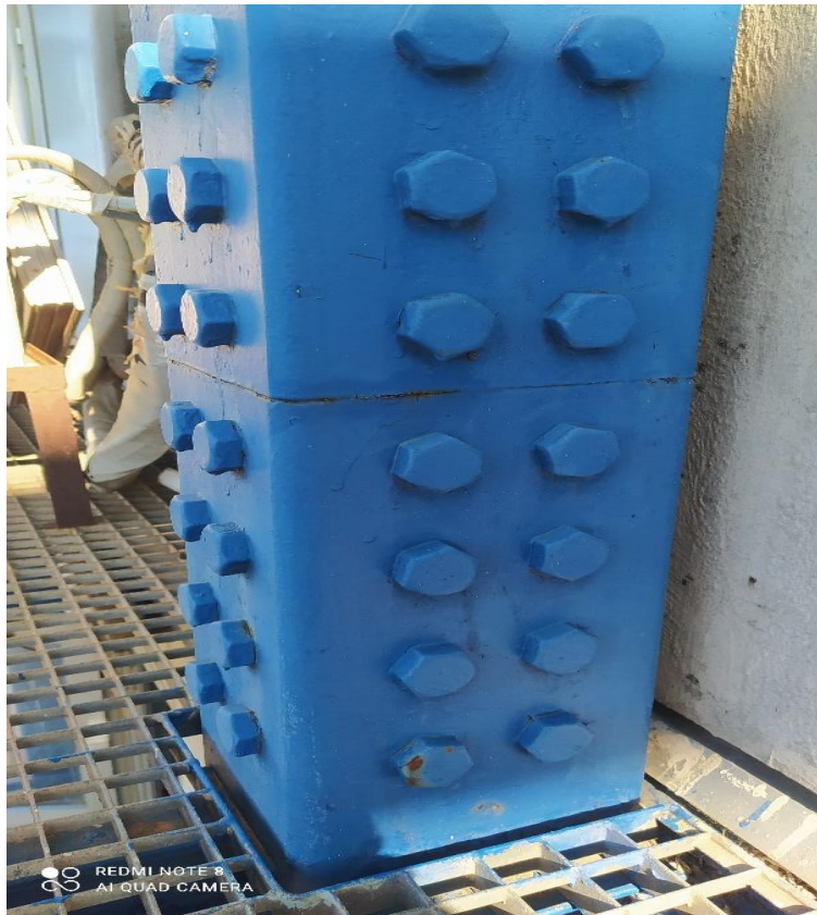
Figure III. 6 : assemblage poteaux-poteaux.
