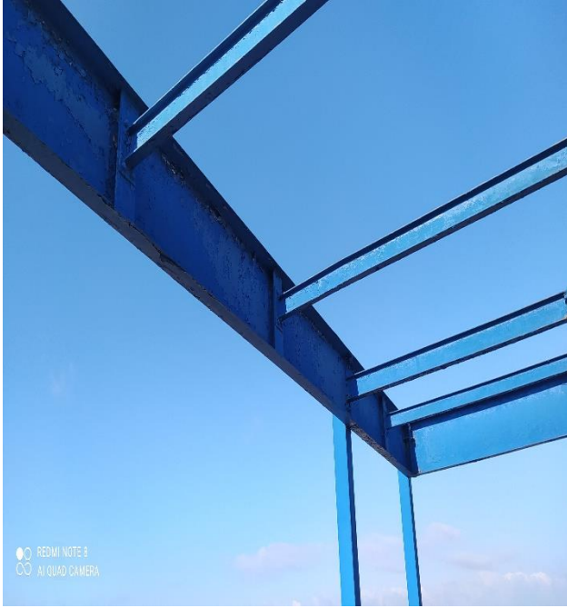
Figure III.4 : assemblage poteau-poutre.
