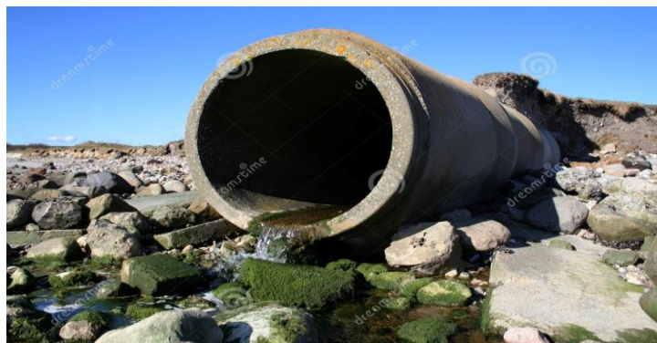
Figure II. 7: le canal d'évacuation 26
