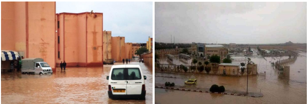
Figure III.6: Les inondations de Djelfa le 08/09/2015
