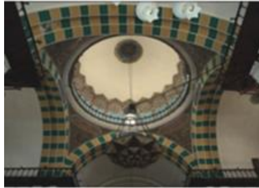
Figure 32. La coupole de Djamaa Djadid.
