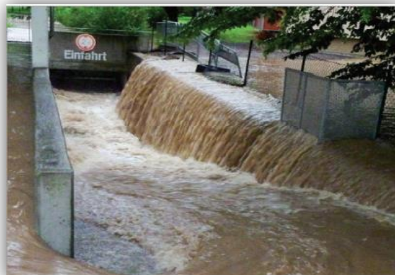
Figure 93: Inondation d'un parking souterrain.
