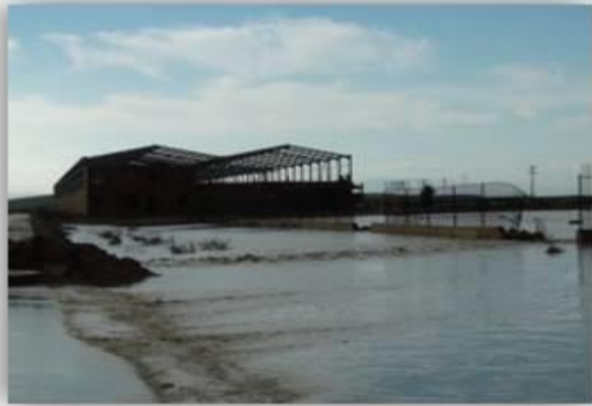
Figure 36: fermeture de la rout. Source: direction d'hydraulique
