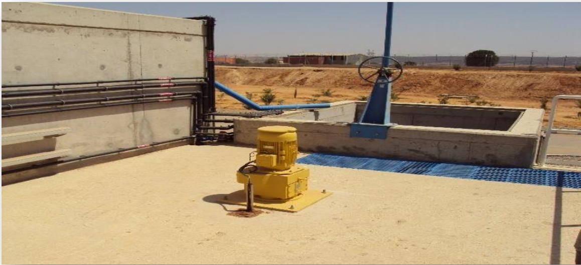
Figure I.8 : Agitation Rapide (Coagulation).
