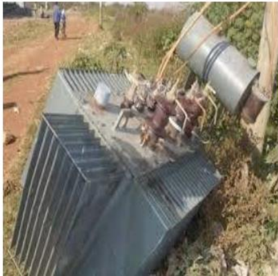
Figure 2. 2:Transformer fall
