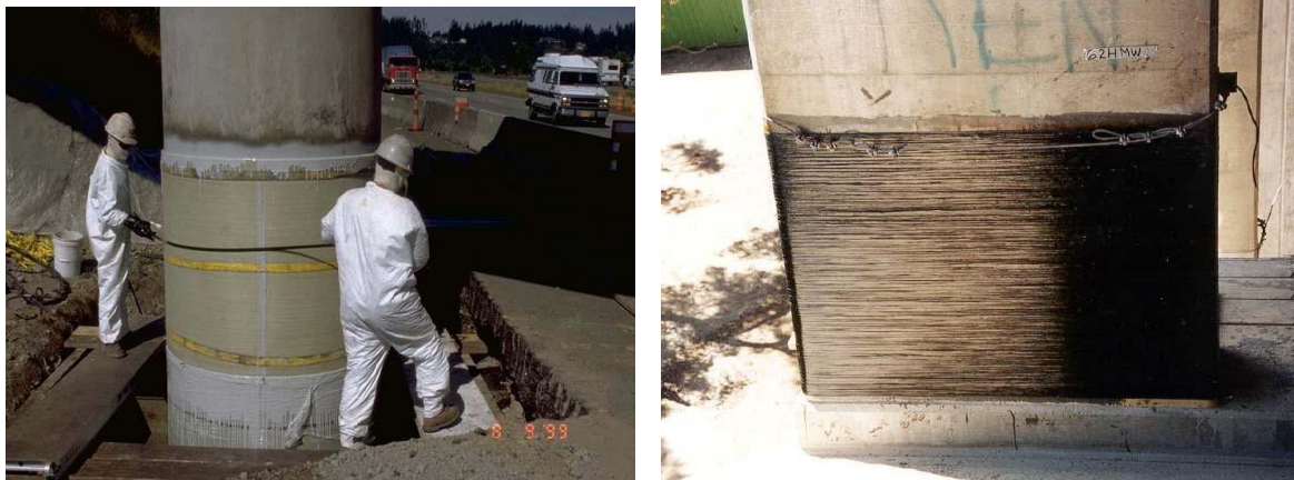
Figure 1.8. Containment of bridge columns by composite materials
