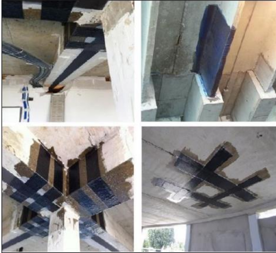
Figure I-11: Several uses of the EBR reinforcement technique (Teng et al. , 2002).
