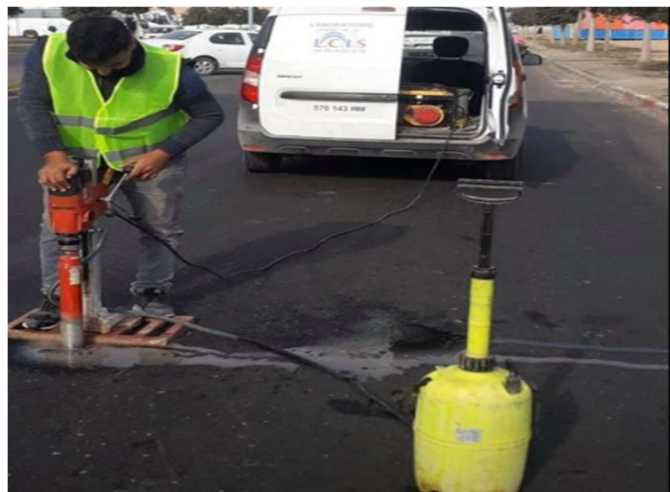
Figure 11-14 essai de carottage
