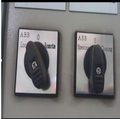
Picture IV.15 : KK and QK selector switch
