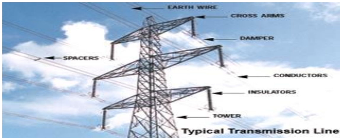
Picture I.2 : Overhead transmission line tower with components.
