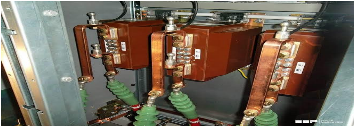
Picture II.26 : Potential transformer measuring circuit.
