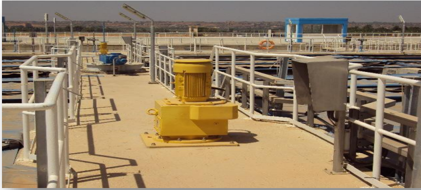
Figure II.9: Agitation lente (floculation).
