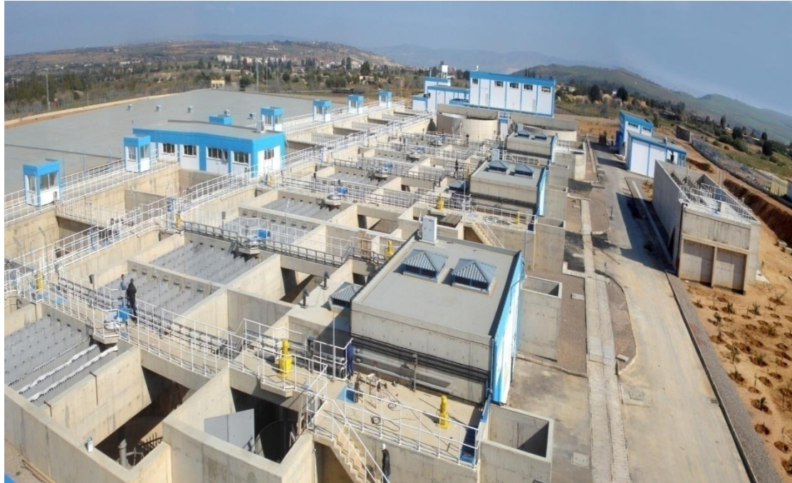
Figure II.2 : Station de traitement d'eau potable «SEOR».
