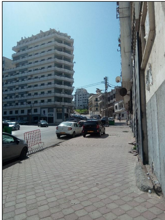
Figure 62. Rue Belhocine (Source : Asma Rezk-kallah, 2019)
