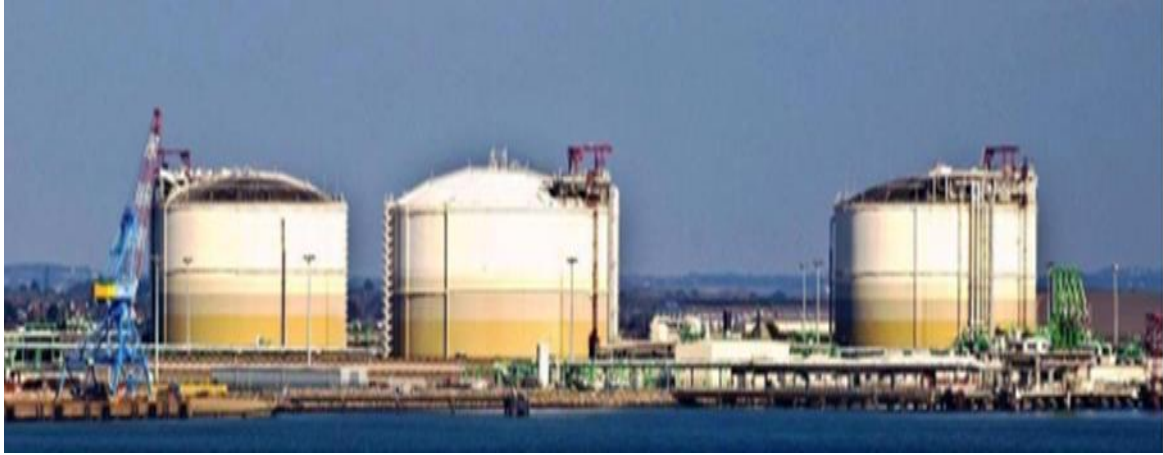
Figure I -4: Bacs de stockages
