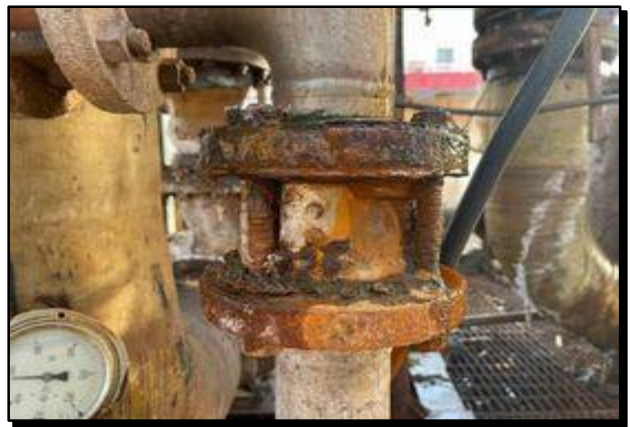
Figure III-11 Corrosion des installations
