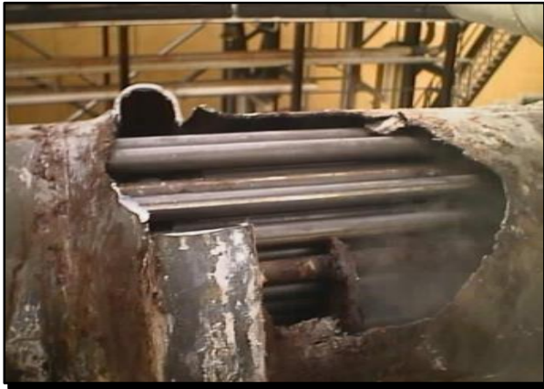
Figure III-11 Corrosion des installations
