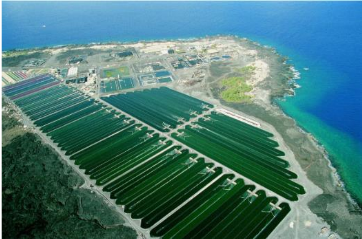
Figure II.14: Exemples des bassins ouverts de type raceway (SCIANDRA.2020)
