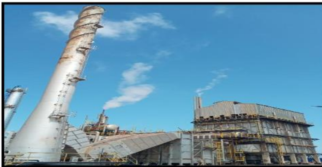
Figure X:Le four de reformage F201(photo prise le 22/03/2023) [1]
