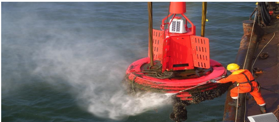
Figure III.8: Cleaning a buoy aboard THV Patricia
