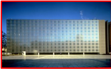
Figure 150: la façade sud
