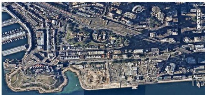
Figure72:photosatellite de site Source: Google earth 2015
