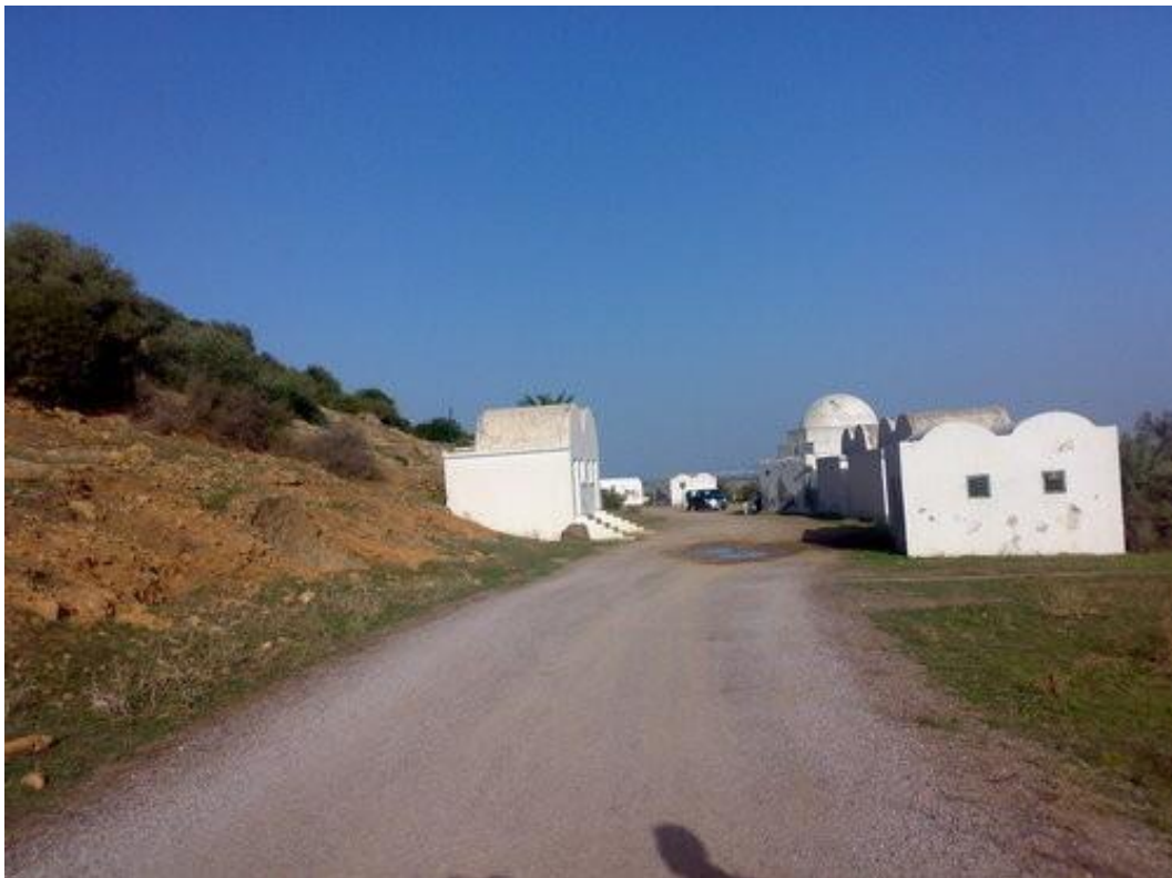
Figure 6: les bains thermaux d Ichkeul. source : Google image
