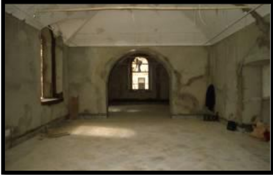
Figure 6 Dar LASRAM avant la restauration
