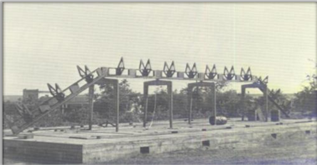
Figure 15: Maison Tropicale (Structure)
