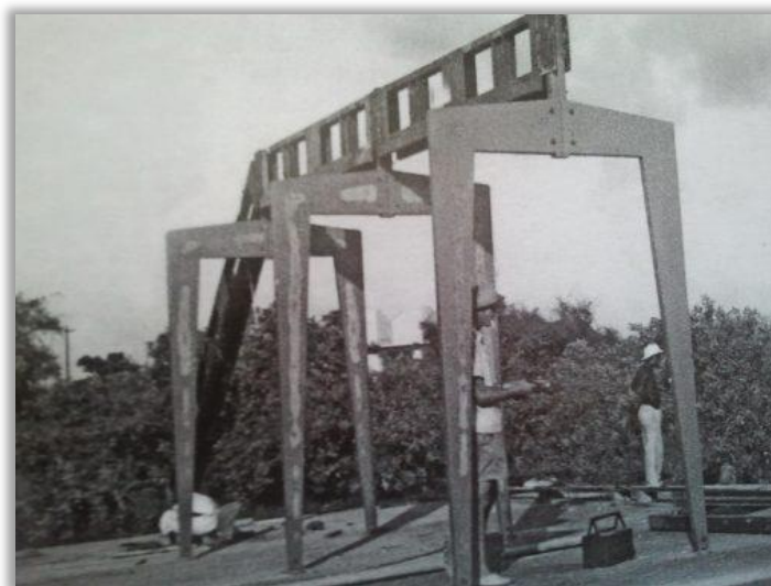
Figure 14: Maison Tropicale (Structure)
