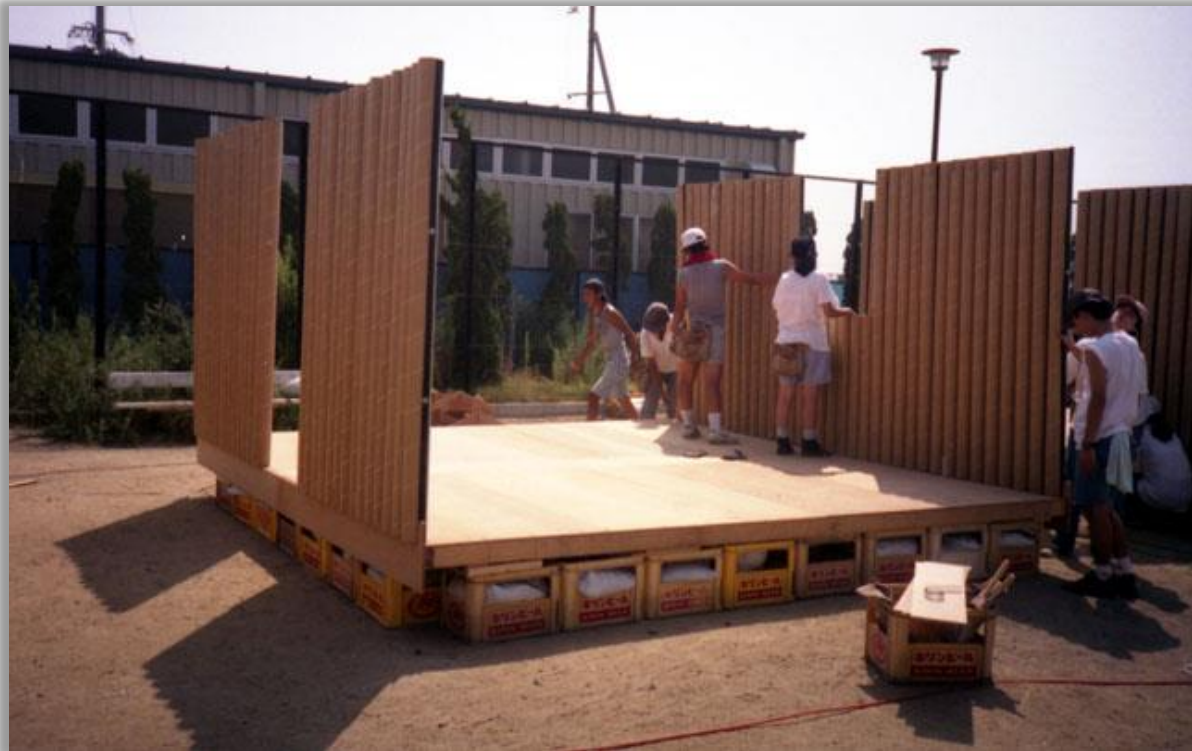
Figure 7: la construction de Paper Log House (1995)
