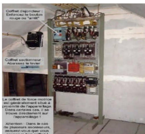
Figure I- 13 : Coffret de force motrice.
