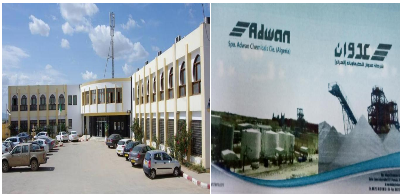
Figure I.1: ADWAN Chemicals Industries Company (ACIC), Algeria
