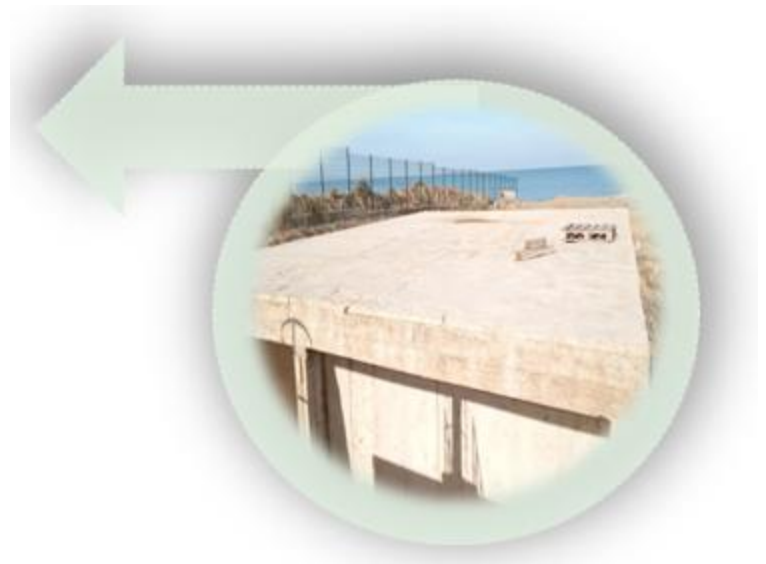
Figure23 :station d'épuration du complexe, Source: SK YSCRAPER CITY.
