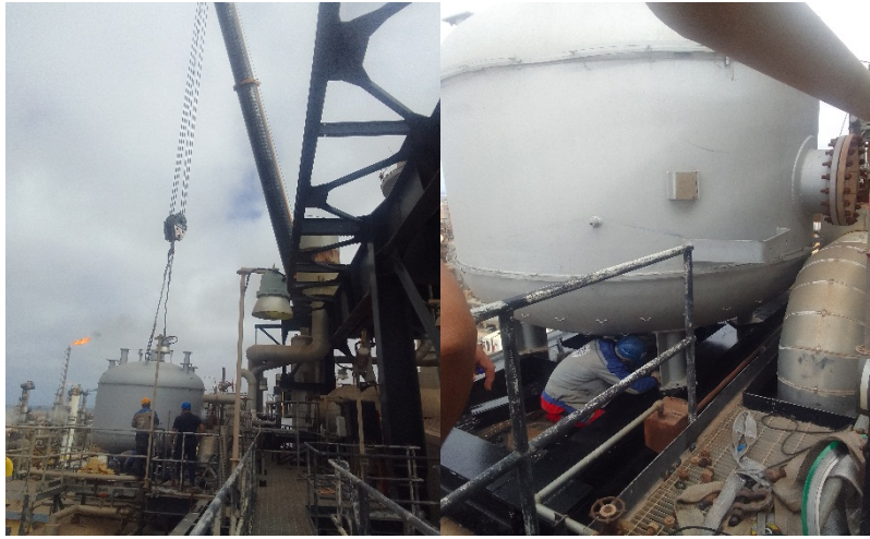
Figure IV.14 : manutention et installation
