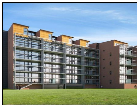
Figure 54 : Tila housing bloc
