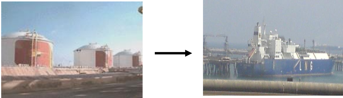
Figure II.7: stockage et transport
