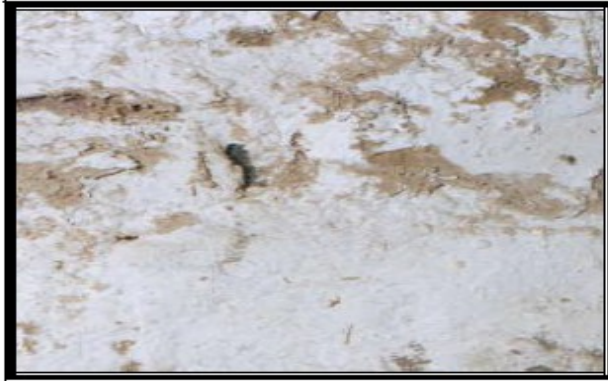
Fig.1.20 : Efflorescences.
