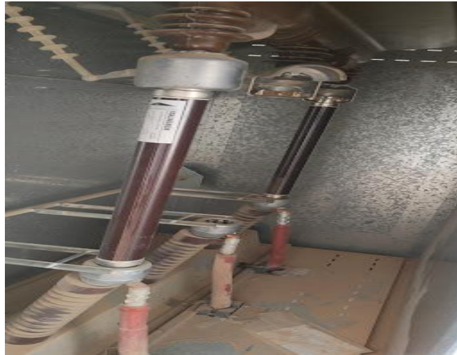
Figure II.41 : fusible MT
