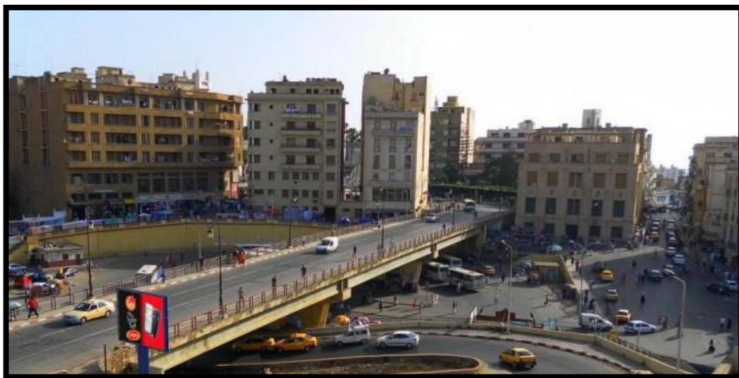
Figure 86: Pont de Ain Safra.
