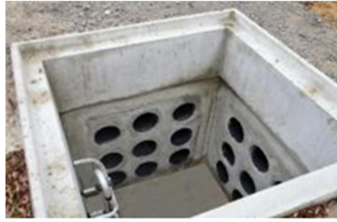
Figure 4.12 :La multitubulaire.
