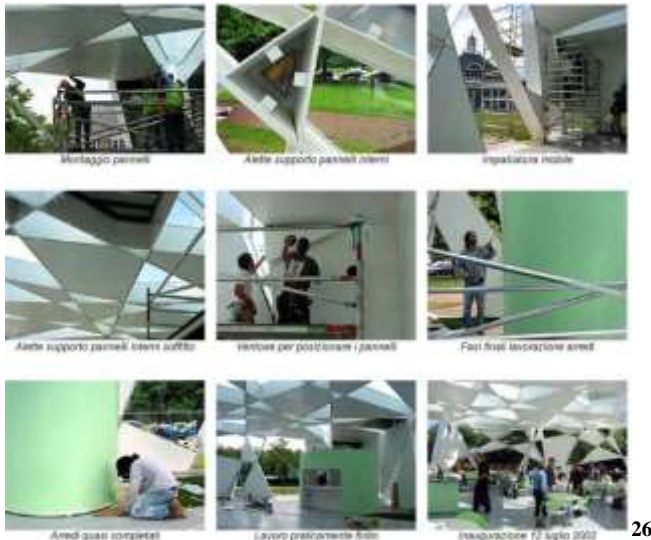
Figure 128: PHASE 4 de construction de pavillon
