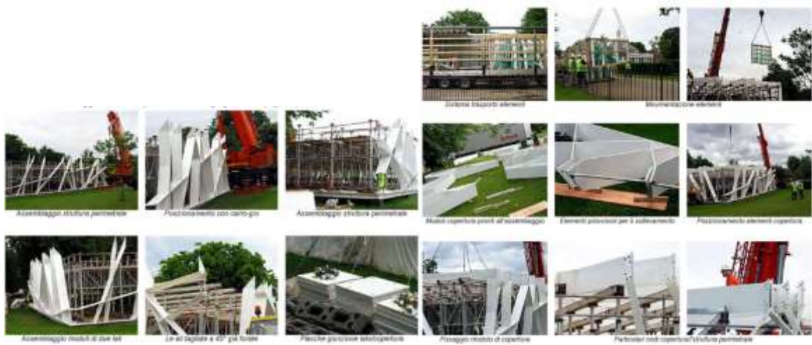
Figure 127: PHASE 3 de construction de pavillon
