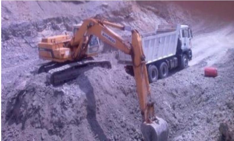
Figure II.3: Chargement et transport.
