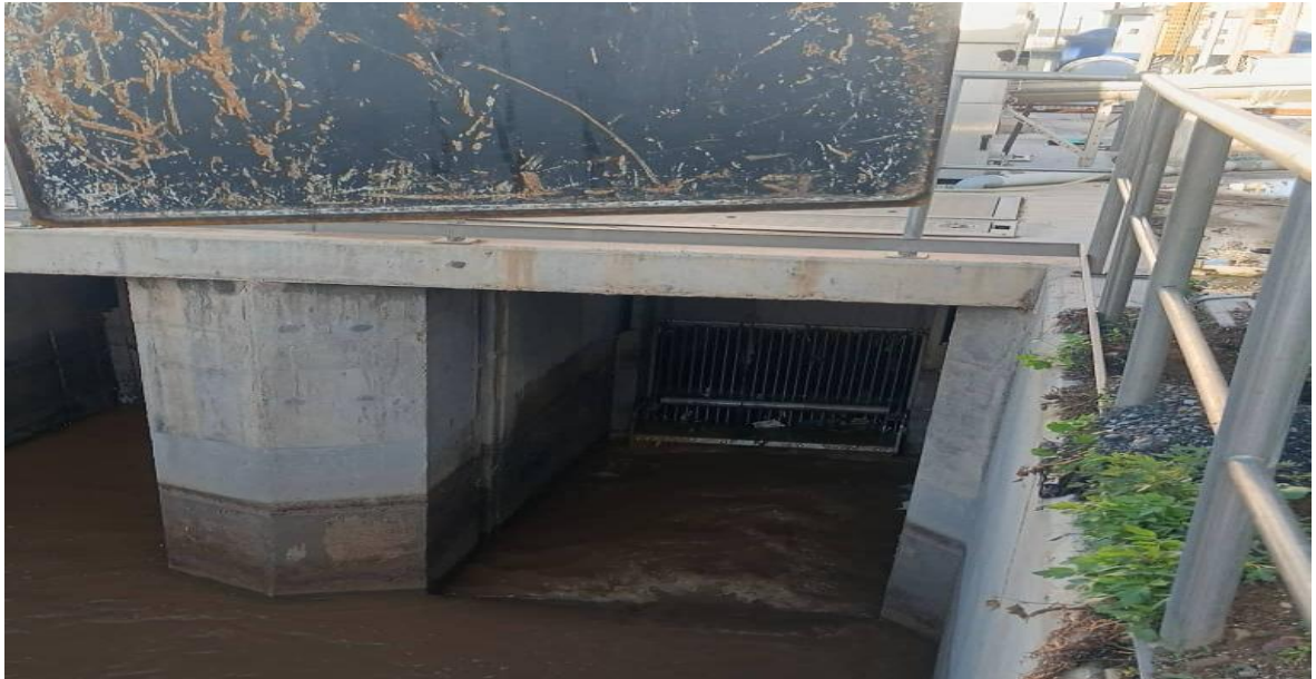
Figure III.05: Coarse screen
