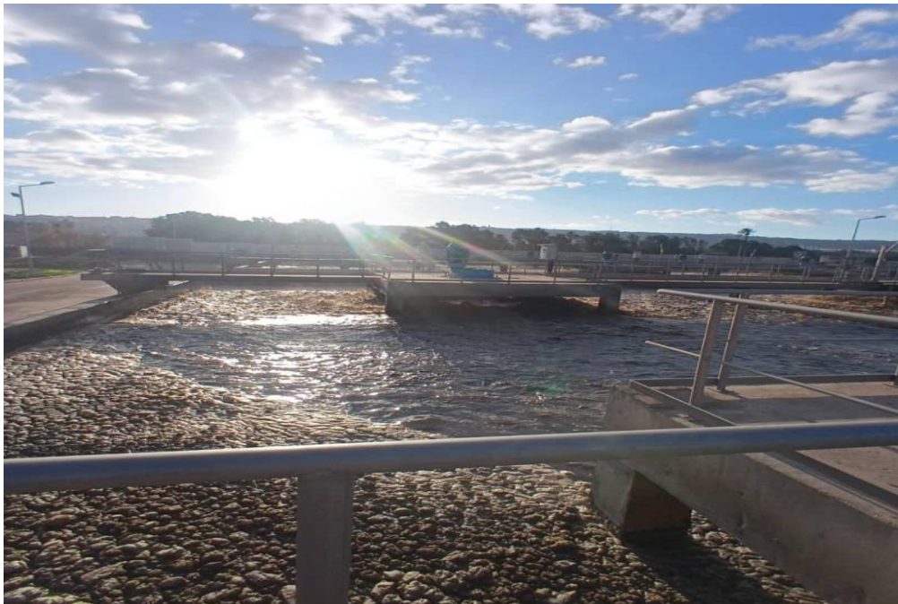
Figure III.07: Biological tank (Aeration tank)
