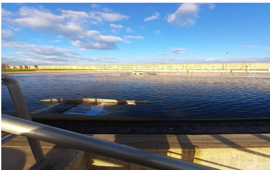
Figure III.08: Secondary clarifiers
