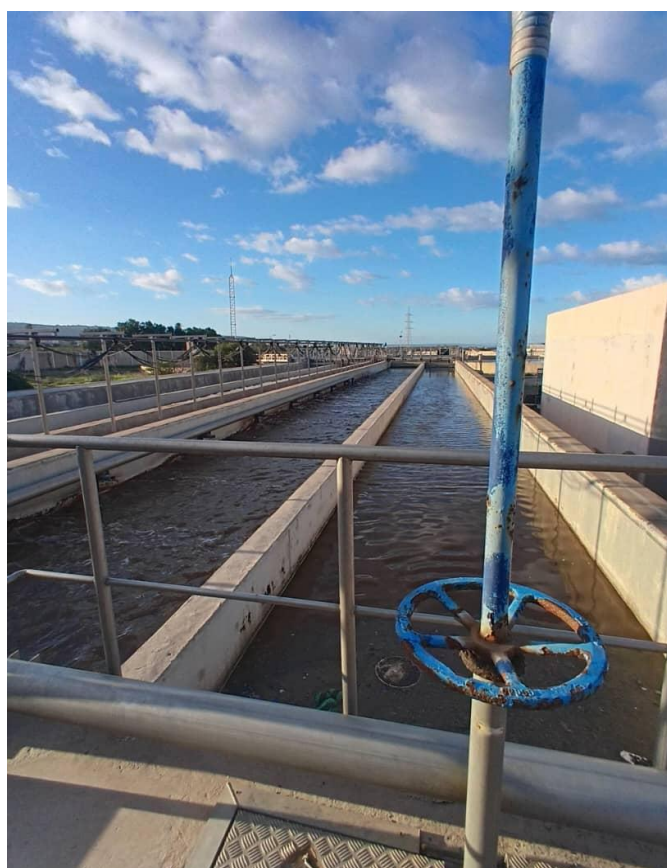
Figure III.06: Desanding and De-oiling
