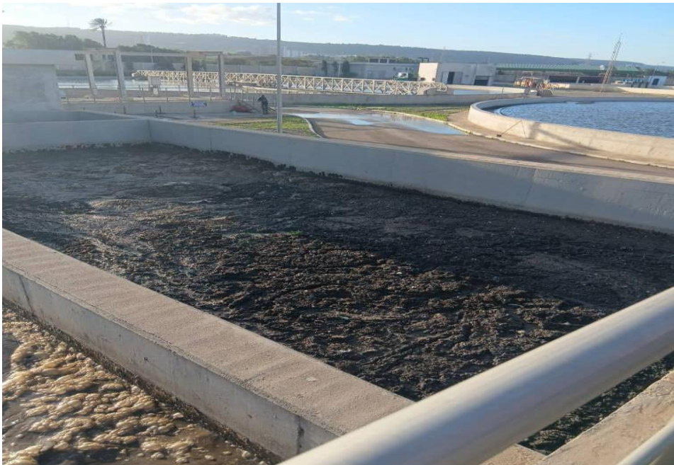
Figure III.10: Stabilization tank
