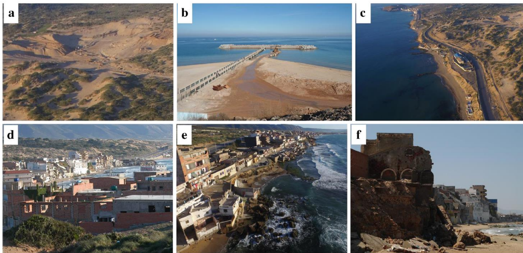
Fig. 10 Human impacts on the sandy coastline of Falcon Cape. a Sand extraction (Sandpit). b Accosting quay and breakwater. c Road network and groins. d and e Urbanization of the dune-beach system. f Coastal erosion, wave damages, and building destructions
