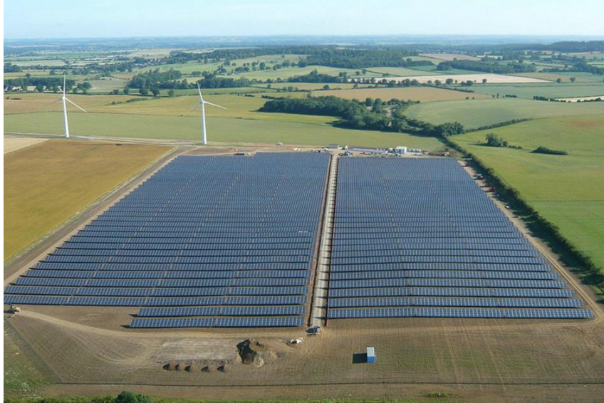
Figure I.20 : station de panneaux photovoltaïques
