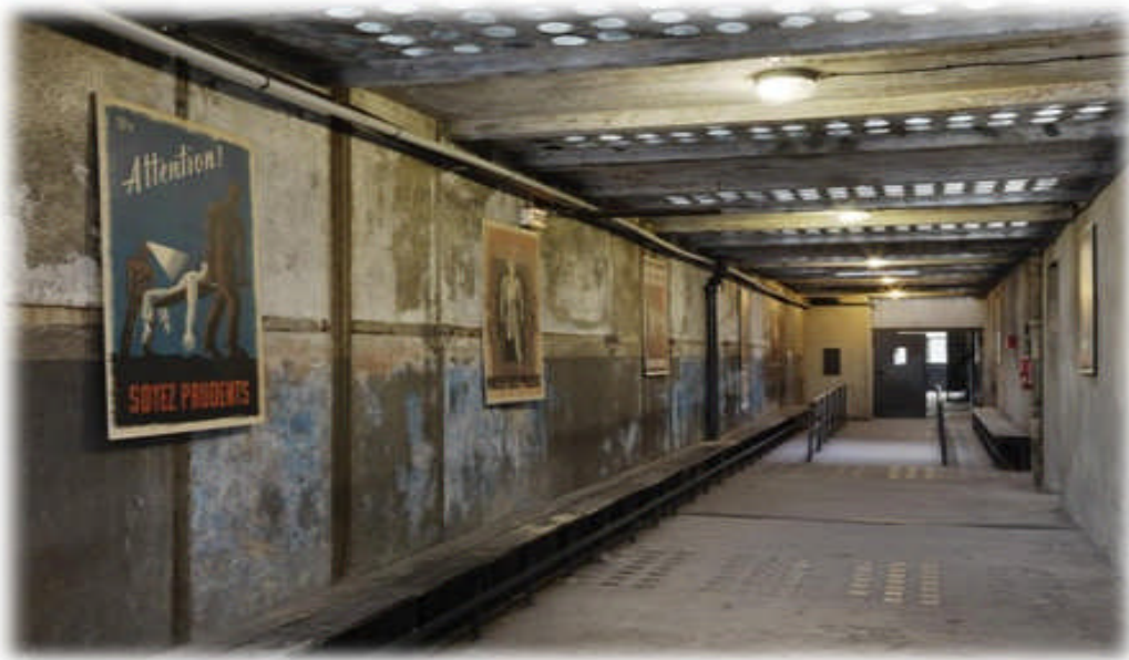
Figure 43 : Couloir du grand lavabo © Florian Kleinfenn
