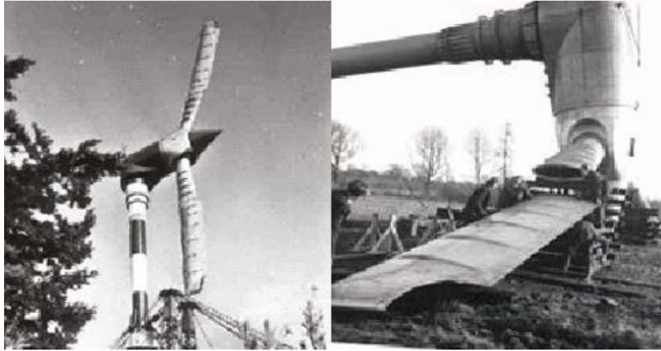
Figure 2.26. (Grand Vent) 100 kW wind Turbine
