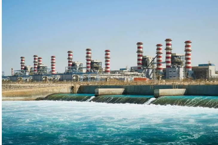
Figure 13: station de dessalement MAGTAA
