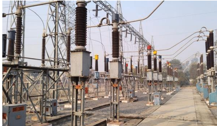
Figure (II.26) transformateur de tension [27]
