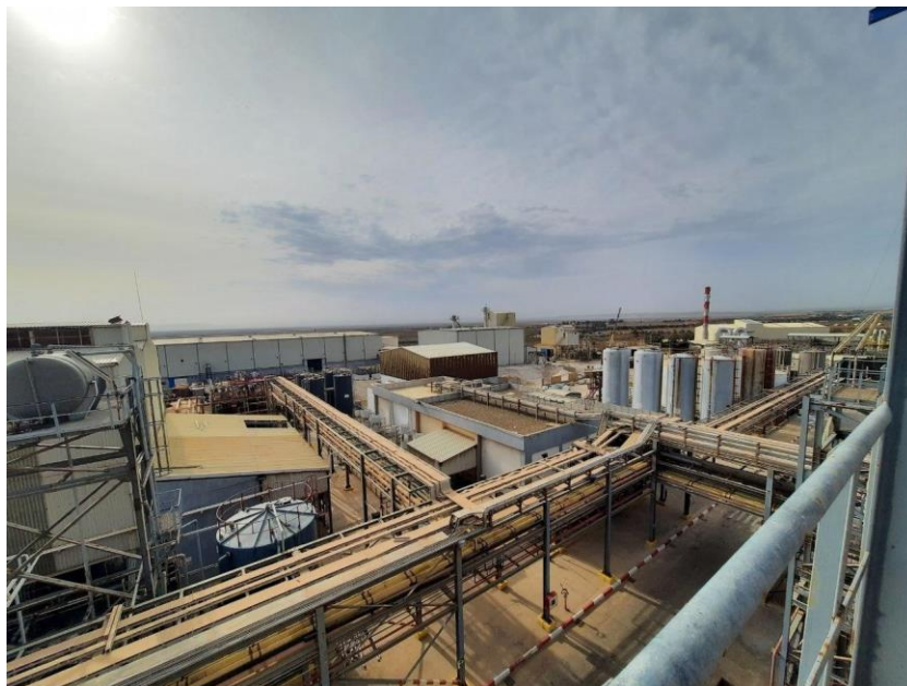
Figure I.1: Adwan Chemicals Algeria
