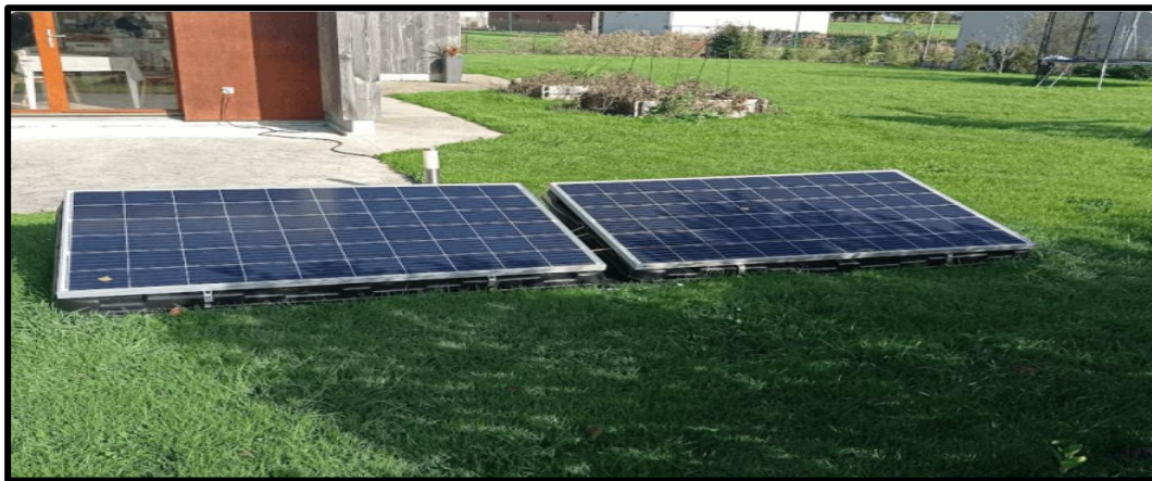
Figure I.15: Ombrage panneaux solaire.
