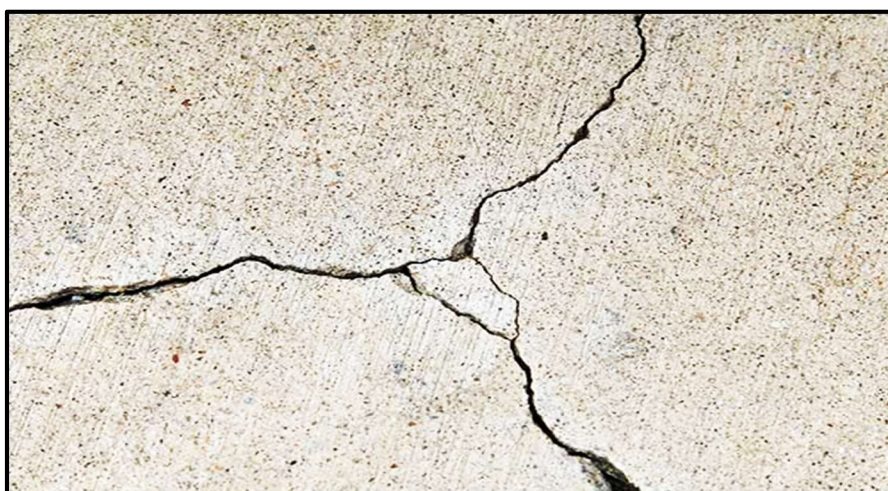
Figure I.10 : Fissures
